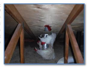
**REPAIR NEEDED:** The ductwork for the hall bathroom exhaust fan is uninsulated in the attic. The ductwork is also poorly installed, and a section of it is undersized. I recommend removing the ductwork from the fan and installing new 4 inch diameter ductwork that is wrapped in insulation as required. All work should be done by licensed professionals.
