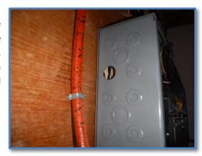
**REPAIR NEEDED:** There are electrical wires in the basement that have been improperly terminated. Even though the wires may not be live, they need to be terminated in an approved junction box, capped and taped so that if they inadvertently become powered they will not electrocute anyone or start an electrical fire. Repair by a licensed electrician is required.
