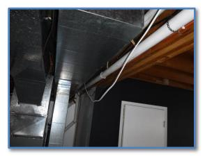
of or beneath framing members, it must be secured to running boards. I recommend that an electrician make corrections as needed.
