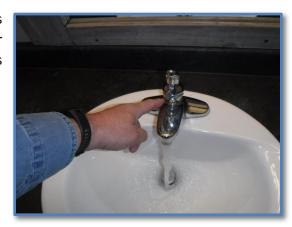
**REPAIR NEEDED:** the faucet at the laundry sink leaks when operated and the laundry tub also has a slow drain. Recommendation: Repair or replacement by a licensed plumbing contractor as appropriate.
