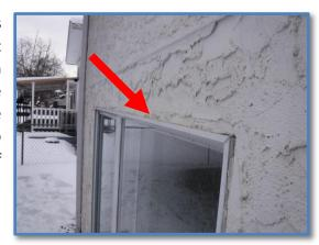
**ATTENTION:** The stucco on the exterior walls of this home is bulging at the floor joist line in one or more locations. This is most likely the result of the floor joists shrinking and drying out causing the stucco to bulge or bow out in the curing process. No repairs are needed unless the stucco cracks. Monitor and repair as needed.
