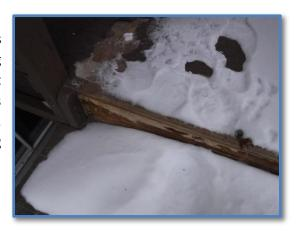
**REPAIR NEEDED:** The handrail for the back deck stairs is not safe as it does not conform to the required safety standards. The required spacing for a railing is no openings greater than 4 inches, and the railing must not
