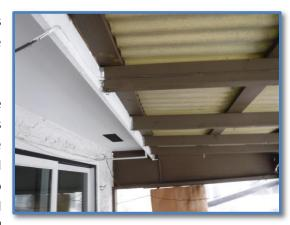
**REPAIR NEEDED:** One or more of the gutter downspout(s) for the home terminate directly next to the foundation. A proper configuration has the downspout(s) terminating at least 6-feet away from the foundation. Recommendation: Repair as appropriate.
