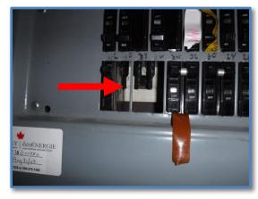
**REPAIR NEEDED:** There are breakers/fuses in the service panel that are rated for more than their associated circuits require. This is known as overfusing. Overfusing can allow more loads on a branch circuit than the wiring is rated for, overheating conductors and leading to electrical fires. The breaker in this case, is associated with the dryer circuit. Recommendation: Repair as appropriate by a licensed electrical contractor.
