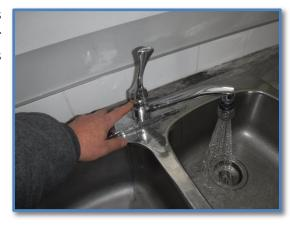
**REPAIR NEEDED:** The faucet at the hall bath sink leaks when operated. Recommendation: Repair or replacement by a licensed plumbing contractor as appropriate.
