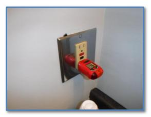
**ATTENTION:** Arc Fault Circuit Interrupter (AFCI) outlets have been required in bedrooms in some jurisdictions since 2005. AFCI outlets protect against circuits overheating. Having a licensed electrician add AFCI protection to the bedroom circuits would be a good improvement.
