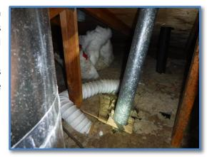
**REPAIR NEEDED:** The exterior walls and ceilings were scanned with an infrared camera in order to determine if areas of insulation were missing or deficient. It was found that there is insulation missing in the attic above one of the kitchen light fixtures. Adding additional insulation to this area is required to prevent heat loss from the home. Have a licensed insulation contractor repair as needed.
